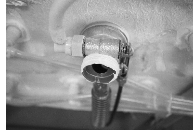
7. Make the thread sealing tape smooth
