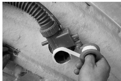
6. Use thread sealing tape to wrap around the drain hole
