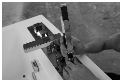
2. Put the shower head into the bathtub in right position as pic. Shows.
